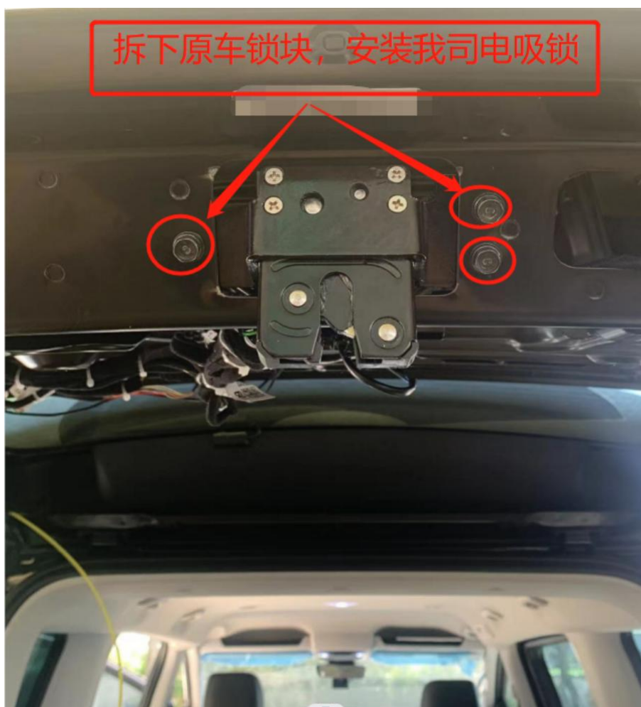
12. Remove the original lock block and replace the electric suction lock.
